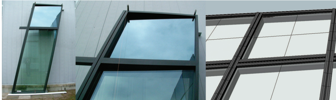
Figure 7.10: Left and centre: facade unit mock up. Right: detail from parametric model.
